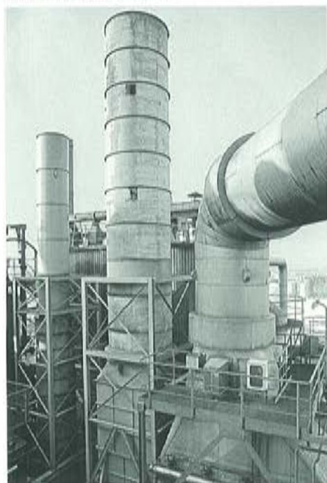
Five metric tons in weight and six meters high: the damper that was fitted to a detergent spray tower in Düsseldorf 1993.
