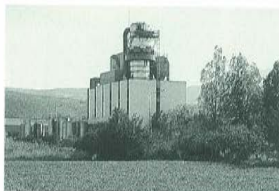
Atalanti: an end-of-stack filter ensures dust-free air.
